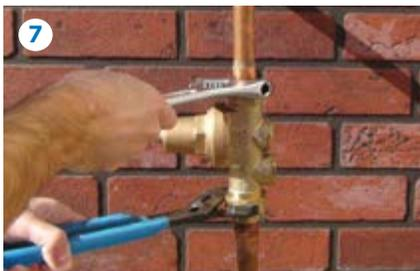
Secure union nut, and use a backup wrench to protect piping. Captured o-ring on body positively seals union connection to 625XL.
