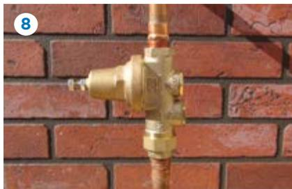
Turn on water to check connections. 625XL is factory set to 50 psi, but can be adjusted as needed.
