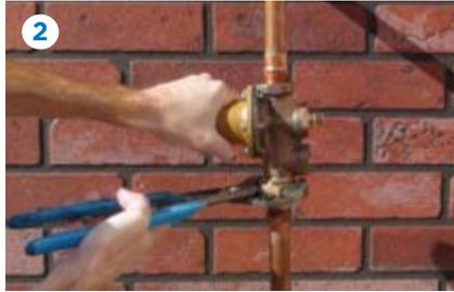
Shut off water and loosen the union nut to begin removal.
