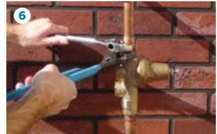
Secure 625XL by using a wrench until tight. Use backup wrench to protect existing piping.
