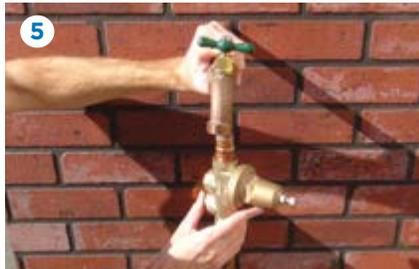
Hand tighten the 625XL onto piping. 625XL exactly matches competitor footprint for easy installation.
