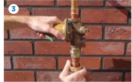
The union nut from previous installation can be used for 625XL installation to reduce installation costs and speed installation.
