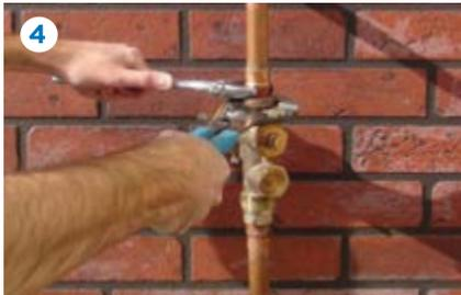
Wrench existing PRV free while using a backup wrench to protect existing piping. Apply Teflon sealant to existing pipe threads.
