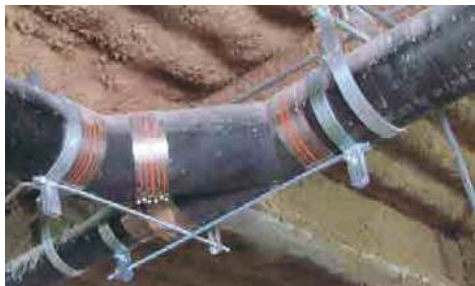
No-Hub Fitting Restraint
