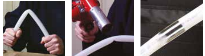
Figure 6-3: Reforming kinked piping
