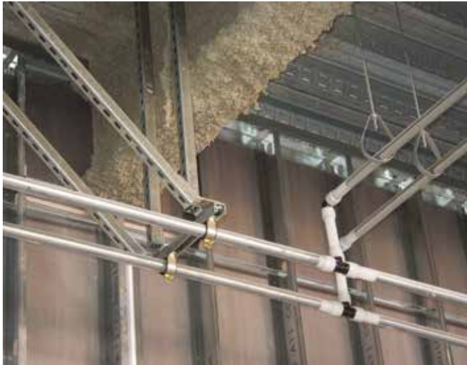
Figure 5-1: Uponor PEX-a Pipe Support
