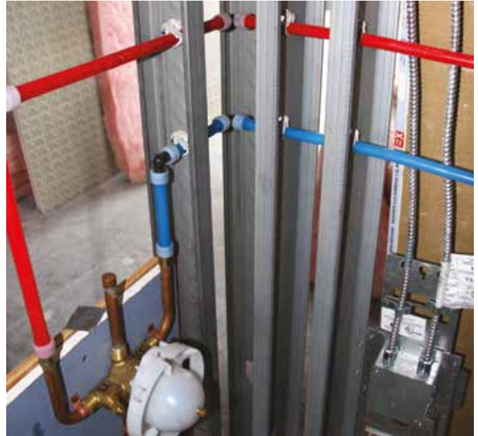
Figure 5-2: In-wall piping
