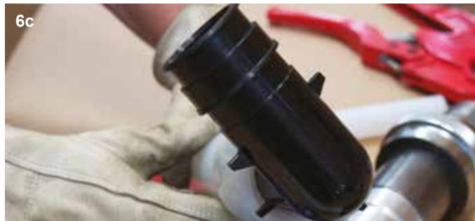
Insert ProPEX fitting into 2" Uponor PEX piping.
