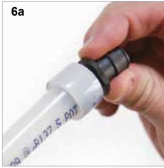
Insert ProPEX fitting into 1/2" Uponor PEX piping.
