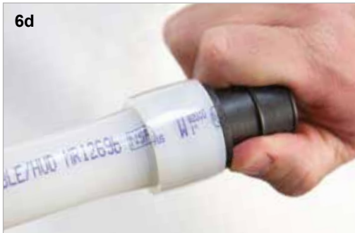
Insert ProPEX fitting into 1" Uponor PEX piping.
