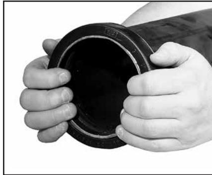
**2 GASKET INSTALLATION**— Slip the gasket over the one pipe, making sure the gasket lip does not overhang the pipe end.
